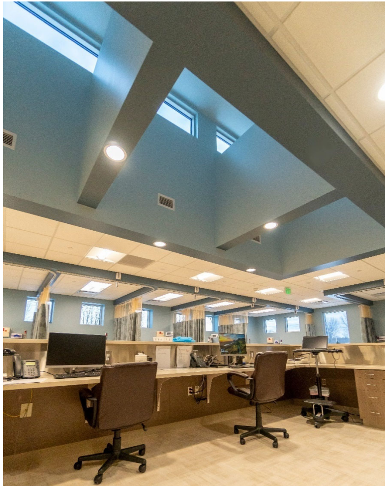
Skylights above the Nurses' Station Provide Natural Light for Staff
