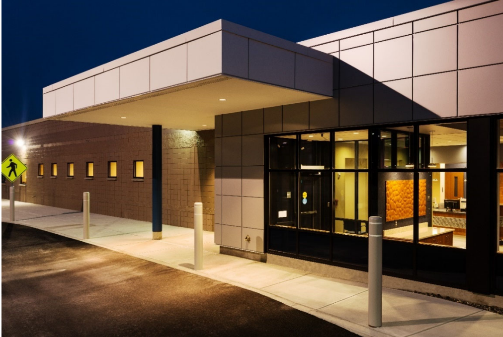
Providing Visual Impact at the front Entry of the ASC While Keeping the Remaining Exterior Walls Simple Can Be a Wise Allocation of Resources
